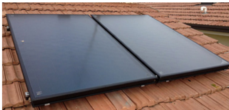
Figure 1: A picture of flat plate collectors (FTP)
